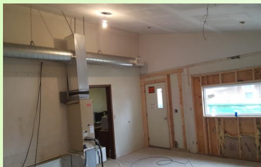
Below: Paneling gone, new window & ducts...
